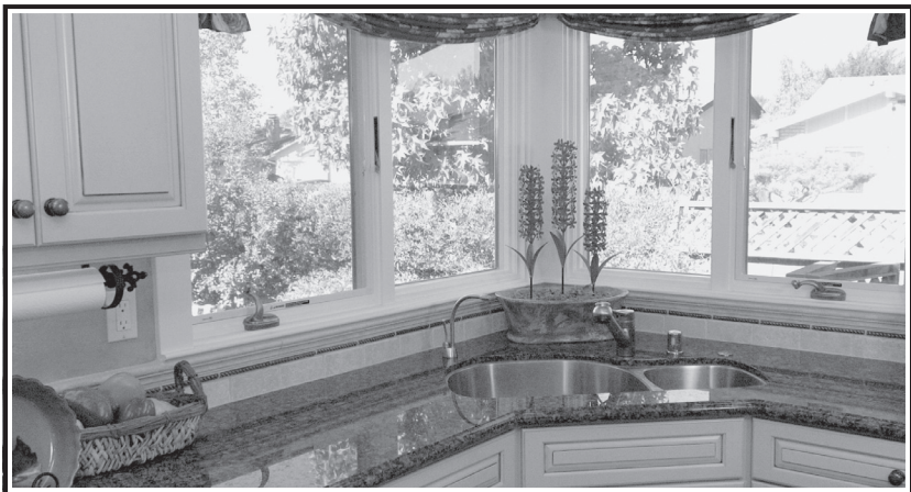
A single row of backsplash with the full splash only behind the range top.
